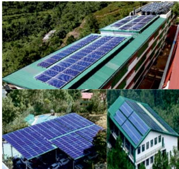
Figure 2: Green Shoolini University township uses a distributed 400kWp grid-connected solar photovoltaic power plant on the building rooftops and car parking to meet the energy needs & reduces dependence on conventional electricity
