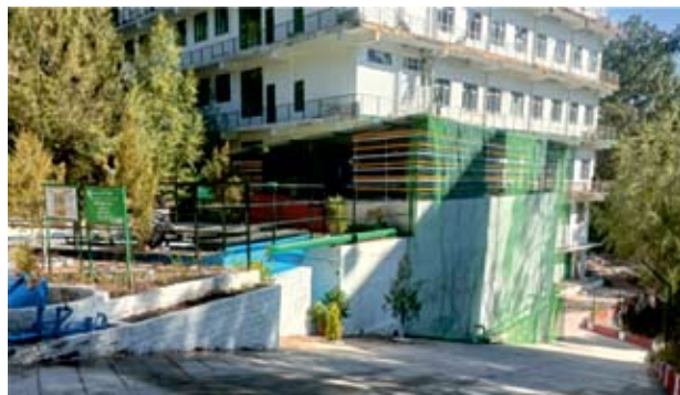
Figure-3: Sewage and water treatment plant at Shoolini University
